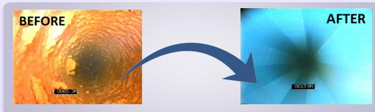
The treatment works directly on the problem, loosening & dissolving the deposits and related contamination. Any of the other standard rehabilitation methods are then used, including surging and brushing, airlifting and pump-in well recycling. Followed by safely pumping the deposits & contamination away.
